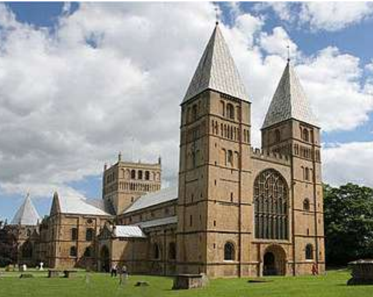
Southwell Cathedral, England
