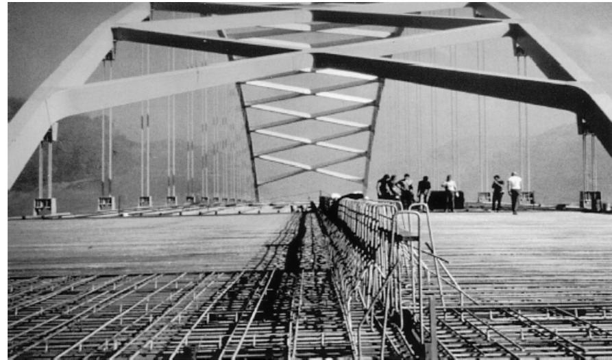
**Figure 5.4 Hot dip galvanized parts and structures prevent corrosion. (Courtesy of Casey Young and Barry Dugan of the Zinc Corporation of America)**
