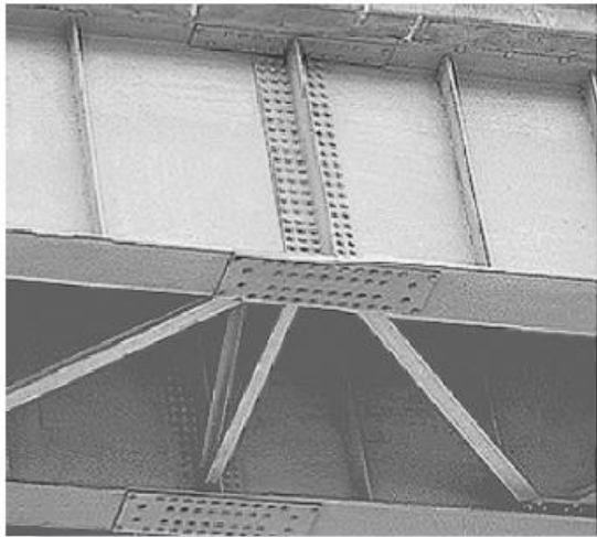
Shown are typical splice plate joints used to connect the steel girders of a highway bridge.
