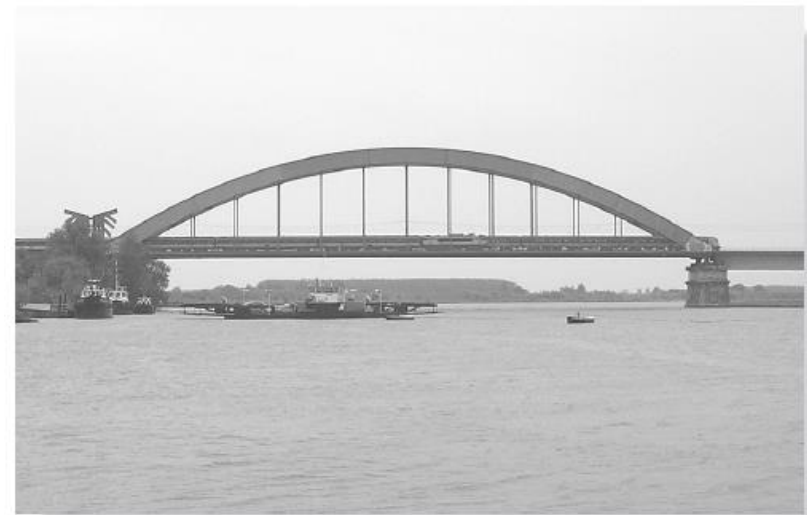
Arches support their loads in compression.
