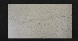
Cracks are necessary for the steel to be used efficiently
