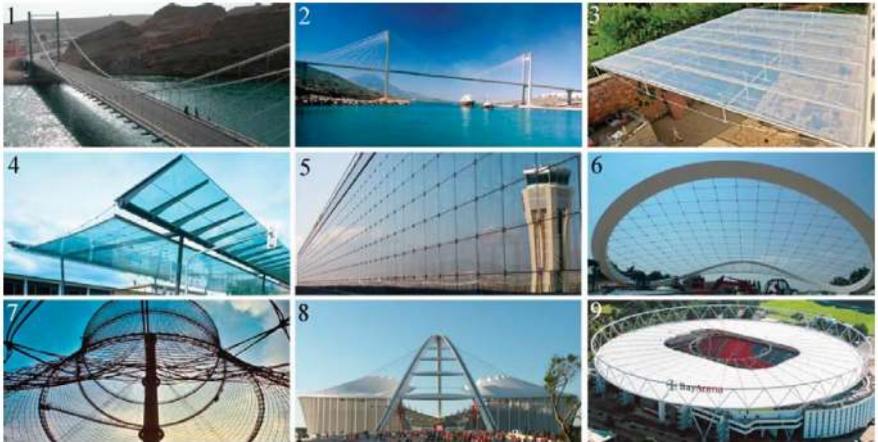
(1) suspension bridge, Highway Bridge Khor al Batah, Oman; (2) cable-stayed bridge, Evripos Bridge, Greece; (3) cable truss roof, Annex Lutherhaus Roof, Germany; (4) cable suspension roof, Glass Canopy of Station Plaza Heilbronn, Germany; (5) cable net facade, Façade Airport Málaga, Spain; (6) saddle-shaped cable net, Canopy in Autostadt Wolfsburg, Germany; (7) cable net tower, Dry Cooling Tower in Schmehausen near Hamm, Germany; (8) arch tower cable supported roof, Moses Mabhida Stadium, South Africa; and (9) spoked wheel cable roof, Bay Arena Leverkusen, Germany
