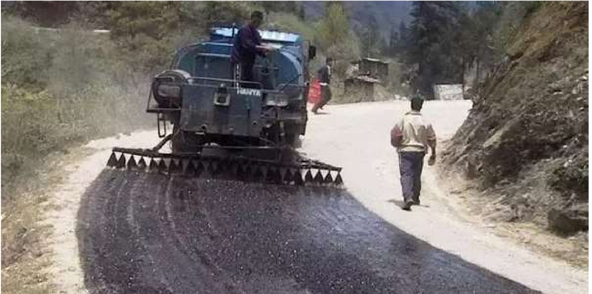
Applying cutback – Prime coat
