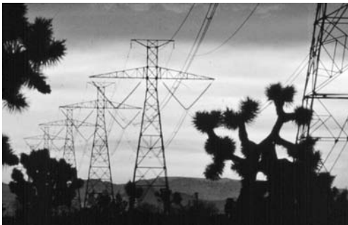
Figure 2 A \pm 500 -kV HVDC transmission line
